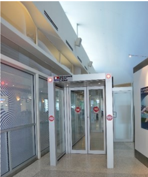
Exit of SEL with closed doors.
