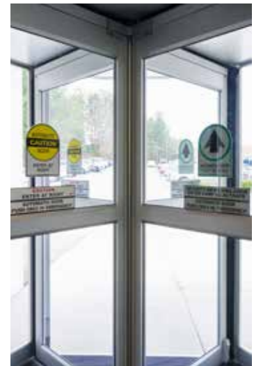
A security revolving door turns one compartment at a time, allowing only one authorized person to enter from the unsecure area.
